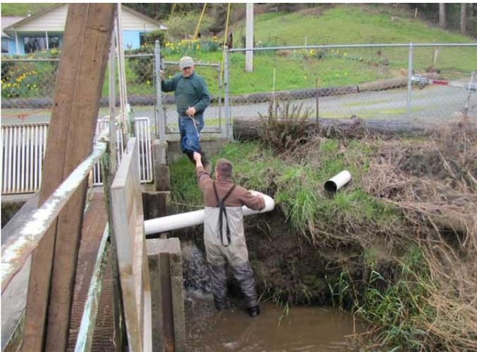
The out flow from Nora's Pond usually goes directly into Noble Creek below the Hatchery. This pipe arrangement below the raceway re-routes the outflow from the pond back into the raceway. This moves the fish from the pond directly into the raceway. That's a lot easier than using nets and buckets to move the salmon.
