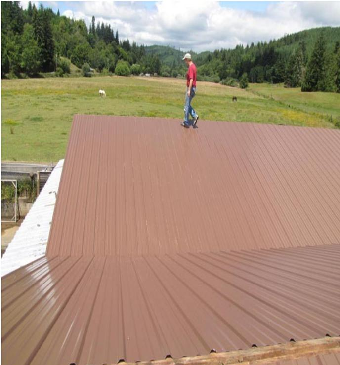
The new metal roof has been installed on the hatchery and raceway buildings. Matt is inspecting the screws on the roof. The roof was screwed down with just enough to hold it in place. It will be finished by another work party in the next few weeks.
