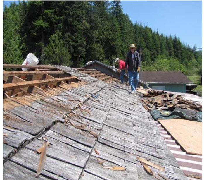
The raceway roof shakes have all been torn off and now the hatchery building roof has to go. Matt and Perk are ripping up shakes and moving them to a trailer to haul away. Bright sun and SPF 45 sun block are the order of the day.
