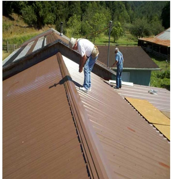
This work party on July 24th is finishing the cap on each roof. A final inspection is also adding screws as needed to make sure the metal is secure and we've done a good job. We are now set for the next rainy season and more salmon to spawn!
