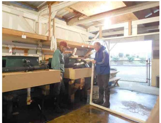
This is the actual installation of the two inch pipe that transports the fry from the hatch box to the holding tank. This is only for hatch box five and six. The fry from the first four hatch boxes output into Nora's Pond. None of the fry are fed in the hatch boxes, only in the holding tanks or Nora's Pond.
