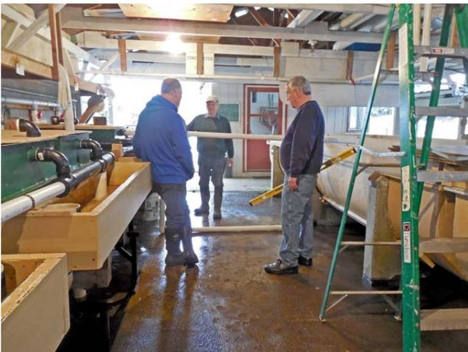
The fry need a way to get from the hatch boxes into the holding tanks. The two inch PVC pipe goes down to the floor then up and over the top of the holding tank. This allows fry to swim out of the hatch boxes at their leisure.
