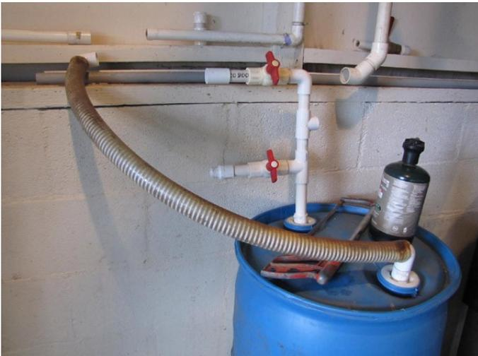
This barrel has been designed by Paul Merz. Its purpose is to help settle out sediment from the water before it goes into the chiller and incubator for our Coho eggs. The rain hasn't brought many Coho but we'll be ready when the rains and Coho arrive.
