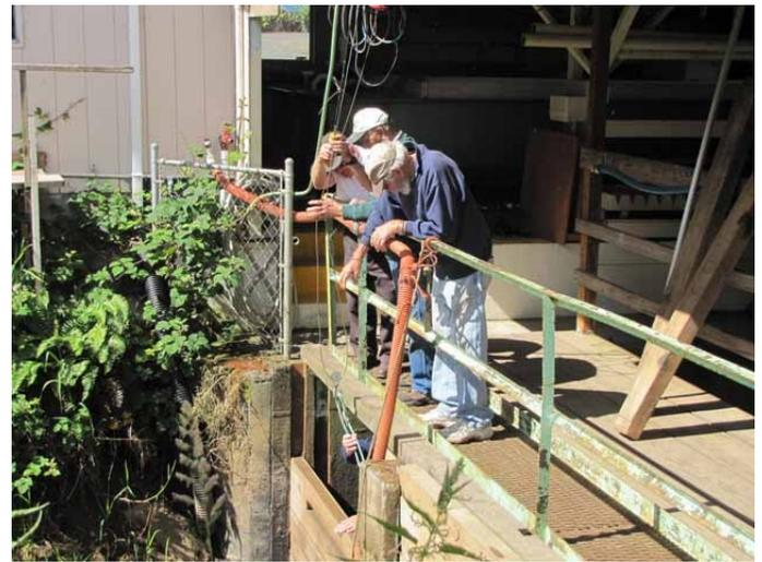
These dam boards have been in place for months. They now come out to be stored for use next year. The electric winch is helpful with some of the lifting.
