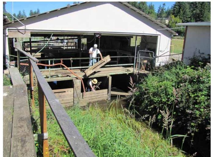
We have an electric winch to help with the heavy lifting. This big 4" x 12" board is the heaviest. The regular 4"x6" dam boards can be moved by hand. We will leave three dam boards in on the raceway side to direct all the creek flow down the right hand trap side. This is enough flow for Cutthroat in the stream.
