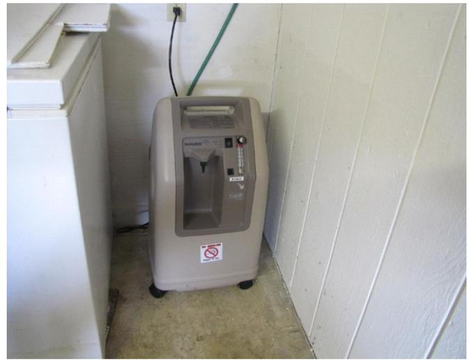
This is the oxygen separator that is being installed by Tod Jones of Redd Zone on March 4th. It removes the nitrogen from air and delivers the remaining oxygen to the low head oxygenator (LHO) to super charge the water with oxygen.
