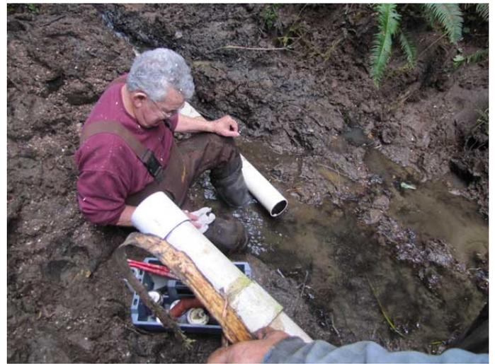
The flow from the upper pond has been getting lower each of the past two years. Harold and Clyde found a spot where the 4" pipe was completely grown over with big willows in the last 30 years. After many hours of shovel and chain saw work the crushed pipe is being replaced with a new heavy duty pipe section.
