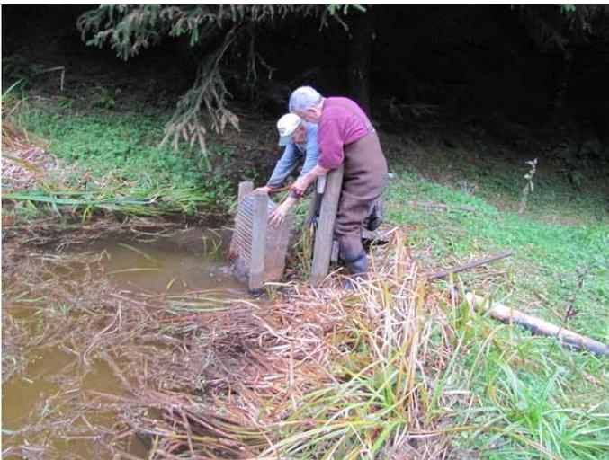
The pond outflow has been blocked off for some time to allow repairs. Now that the new section of pipe has been installed it's time for testing. The stand pipe was removed and the screen installed. The flow at Nora's Pond is about double what it had been before the repairs. **Success!**
