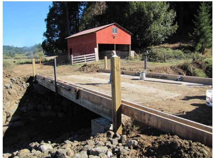
The concrete elements of the bridge are all in place and grout installed to seal between the pieces. Forms are in place for a concrete rail. A 2" x 6" pressure treated wood railing will be installed along each side of the bridge. A gate will also be installed at the far end to keep horses in the pasture. Thank you Coos Watershed for a fine bridge!!!
