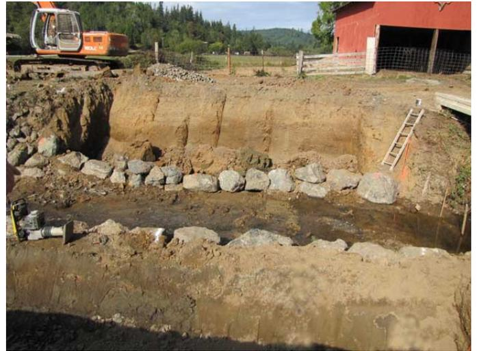
The stream channel has been dug out and a rock base for the creek has been installed. The big boulders are to protect the base of the abutments for the bridge.
