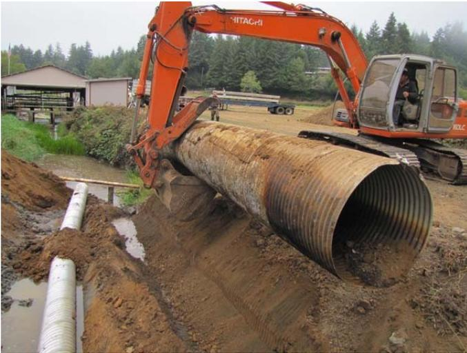
Coos Watershed received a grant to remove the culvert just above the hatchery. It was an undersized culvert which restricted stream flow at high water. A nice big bridge will go in its place.
