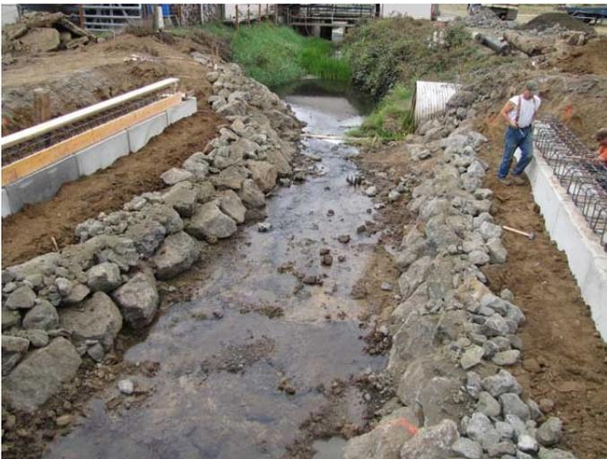
Noble Creek will now have a lot of room for high water events without restricting the stream flow. Concrete footings will be poured on top of the block abutments and the bridge will sit on those. The culvert on the right side of the picture is Ferry Creek entering from the north.
