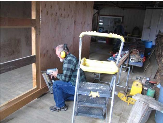
Bob brought his air compressor and nailer to install the 3/4" plywood walls. What a life saver. I'd hate to think how long it would have taken to do it all with a hammer or a screw gun.
