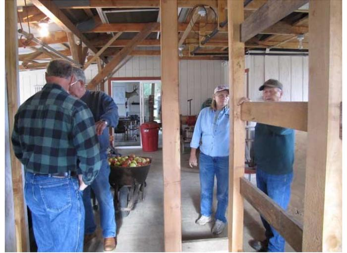
The framing for the walls are from 4"x6" posts on 4' centers. 3/4" plywood walls will be nailed to the posts and 2"x6" horizontal boards. We don't think an earthquake could take it down.
