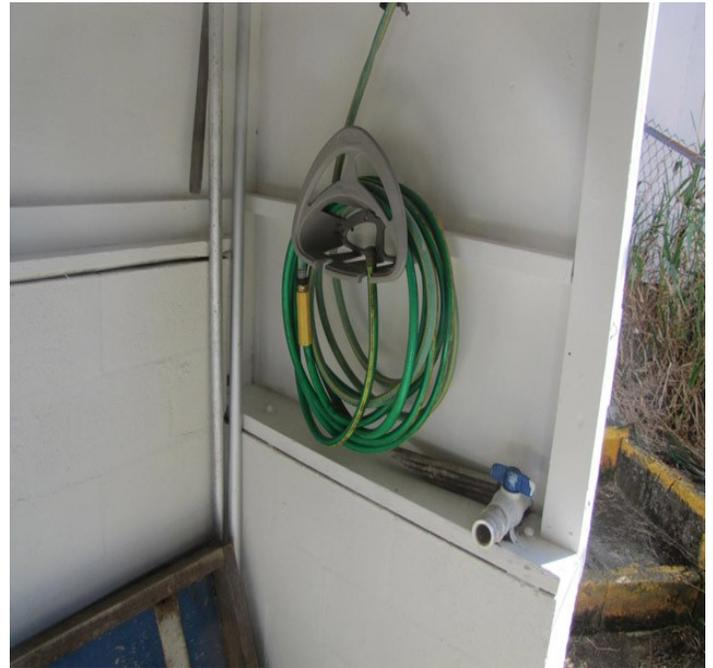
This newly installed hose and rack is next to the table where we cut the carcasses in two. There is a newly installed sump pump and catch tub which will pump things washed off the table out into the pasture behind the hatchery.
