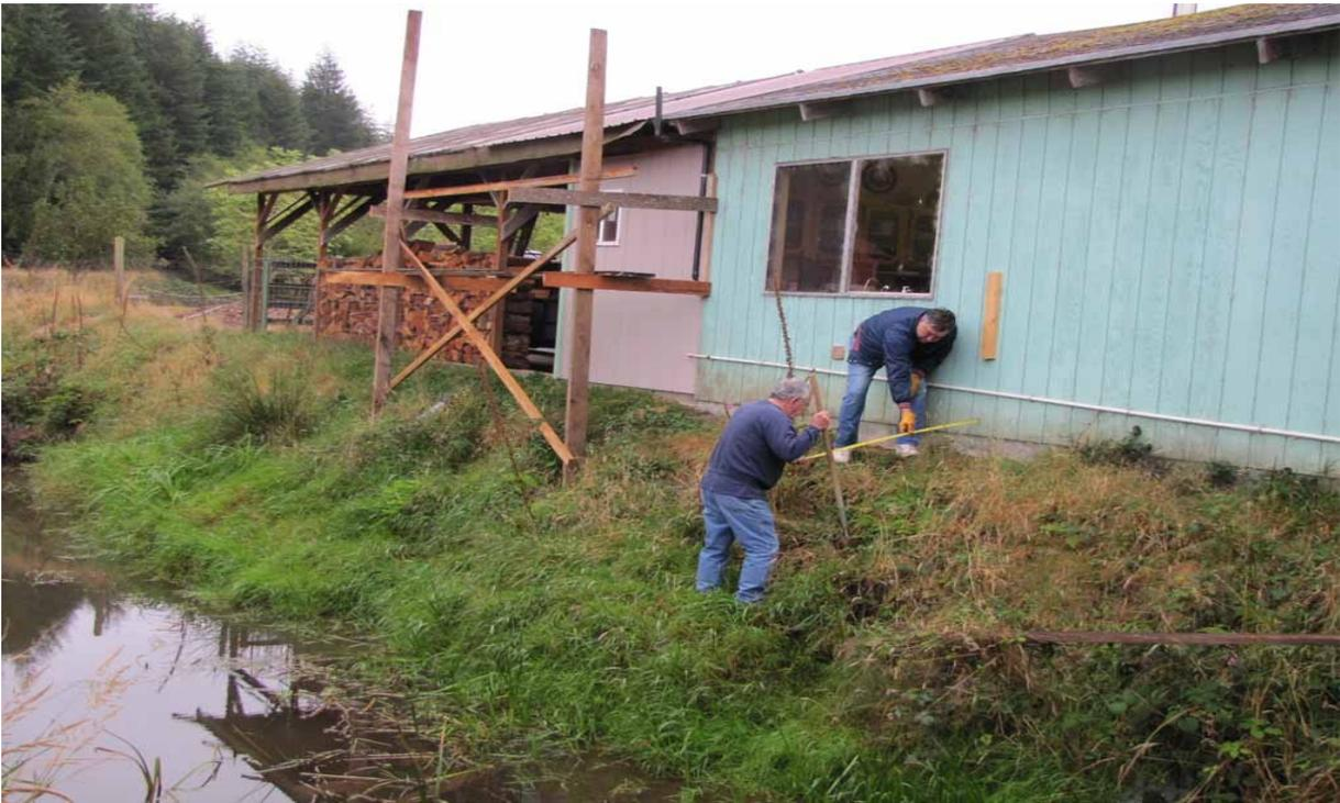
Scaffolding is installed to keep people out of the creek while installing new gutters.
