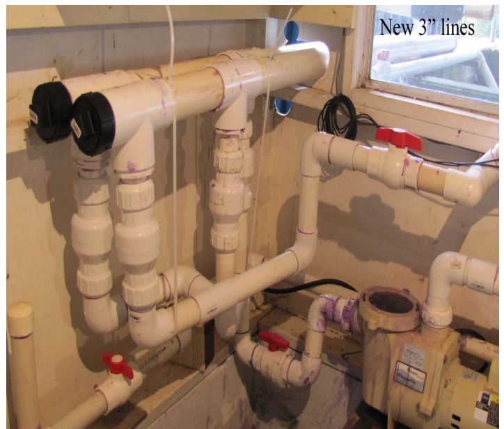
The new 3" lines coming into the hatchery and on to the filters will provide more flow to the hatch boxes and tanks we use to raise our Chinook. The anti-siphon valves allow both water sources to be used. If either source fails the system automatically uses only the one source that's available. Either water source has sufficient flow to handle the water needs for all of our fish.
