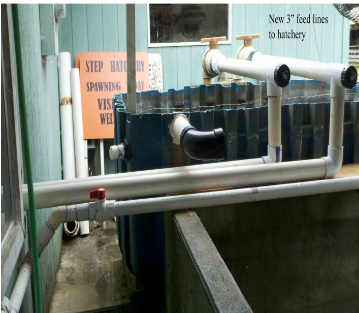
The new 3" lines coming into the hatchery and on to the filters will provide more flow to the hatch boxes and tanks we use to raise our Chinook. The anti-siphon valves allow both water sources to be used. If either source fails the system automatically uses only the one source that's available. Either water source has sufficient flow to handle the water needs for all of our fish.
